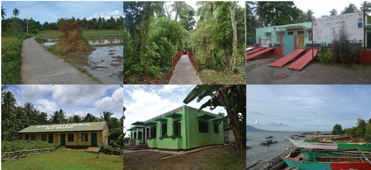
Examples of subprojects under the KC-NCDDP (clockwise from upper left): a pathway in Barangay Catanagan in Juban, Sorsogon; a footbridge in Barangay Calateo, Juban, Sorsogon; a community development center in Barangay Añog in Juban, Sorsogon; a boat dock in Barangay Tulay in Casiguran, Sorsogon; an evacuation center in Barangay Tigbao in Casiguran, Sorsogon; and a school building in Barangay Casay, Casiguran, Sorsogon.
