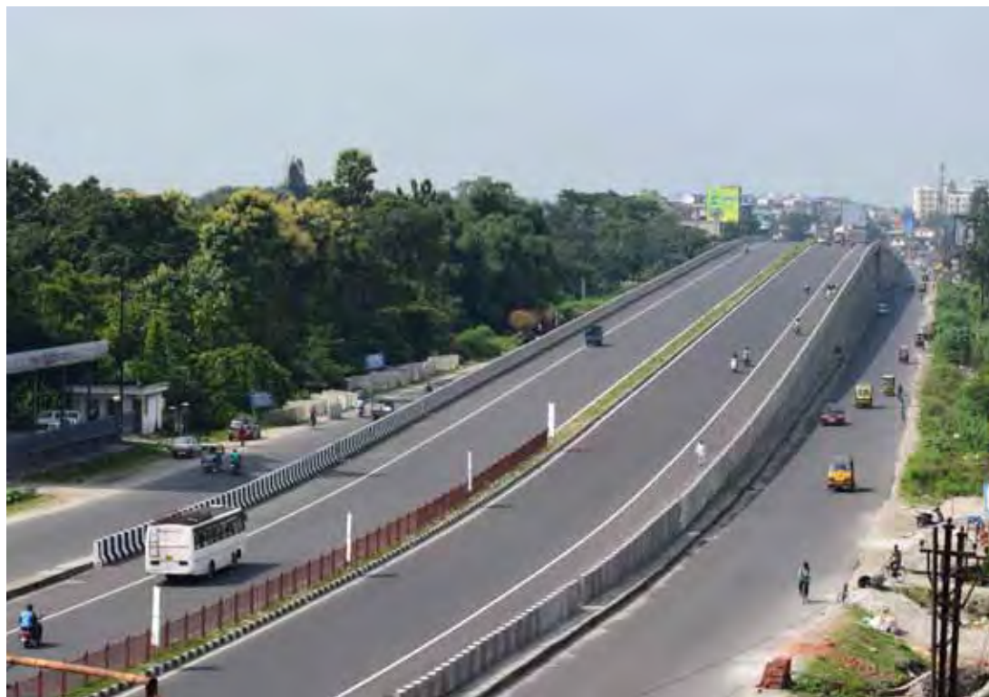
Cross-border connectivity. Road constructed under SASEC Road Connectivity Investment Program, Tranche 1 (photo by ADB).
