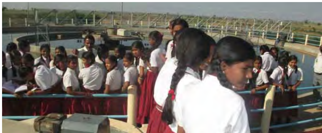
Water close at hand. Students at a water treatment plant in Ilkal, one of the first towns to achieve 24x7 water supply (photo by KUIDFC, Bengaluru).
