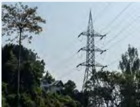
Green corridor. A transmission tower constructed by POWERGRID (photo by ADB).
