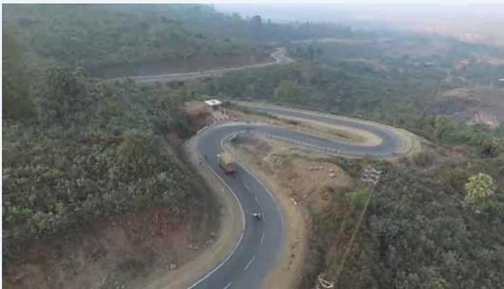
Linking remote regions. A section of the 311-km long state highway built under the ADB-supported Jharkhand State Roads Project (photo by ADB).
