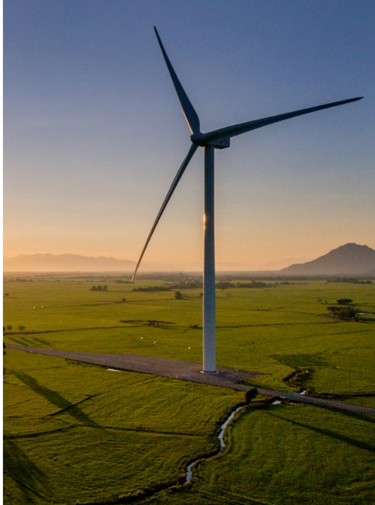
▲ Wind energy. In Viet Nam as elsewhere in the GMS, wind energy capacity is rapidly expanding as it becomes more cost-efficient.
