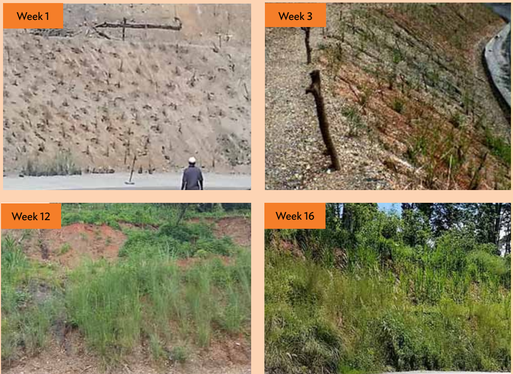
Figure 4: Using Mixed Grasses in Soil Bioengineering
