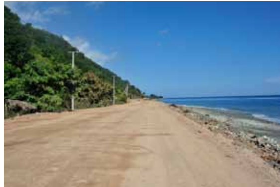
Top: Existing road in Lautem, 2017; Bottom: Existing road in Atabae, 2017.
