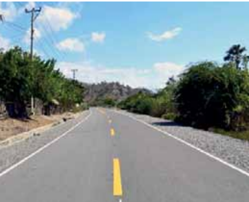
Top: Condition of the section R-4 Km 19+740, as of October 2014; Bottom: Completed road section, 2017.
