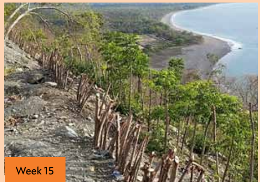
Figure 3: Using Live Stakes Method in Soil Bioengineering
