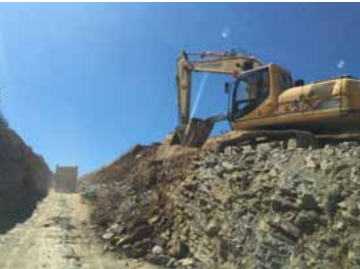
Top: Laclubar Junction, 2017; Bottom: Laclubar bypass construction, 2017.
