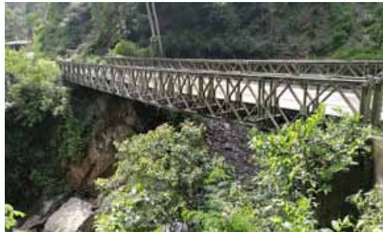
Top and bottom photos: Existing district roads in Ermera district.
