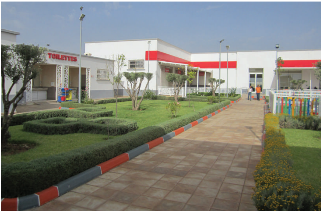
Rest area in a Casablanca–Beni Mellal motorway in Morocco. This rest area provides services such as public toilets, parking, and restaurants. (photo by Ignasi Ragas)
