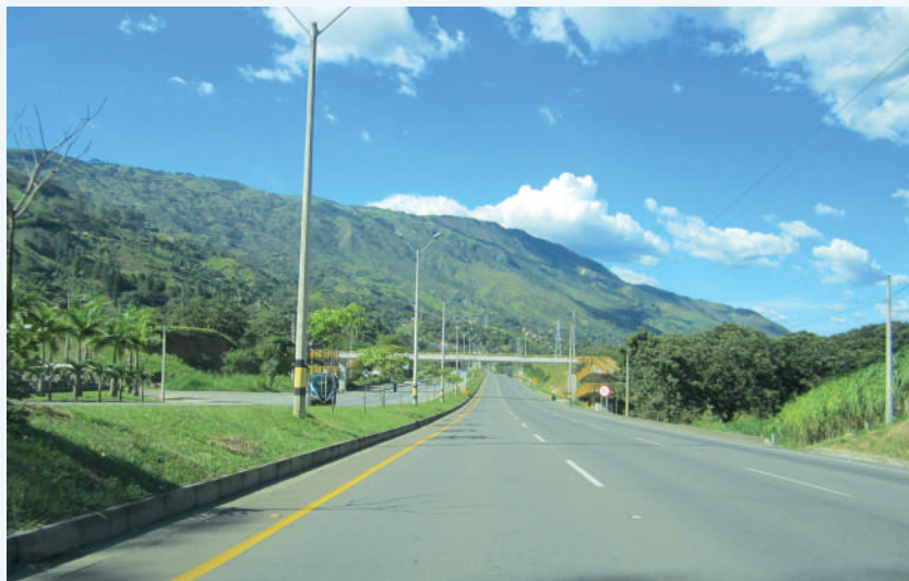
Motorway Medellín–Cartagena. The motorway connecting the cities of Medellín and Cartagena is one of the toll highways in Colombia. (photo by Ignasi Ragas)
