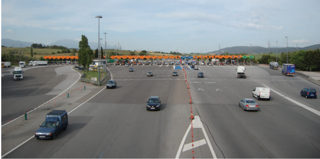
Toll plaza in Spain. Many motorways in Spain are subject to distance-based toll charges. (photo by Ignasi Ragas)
