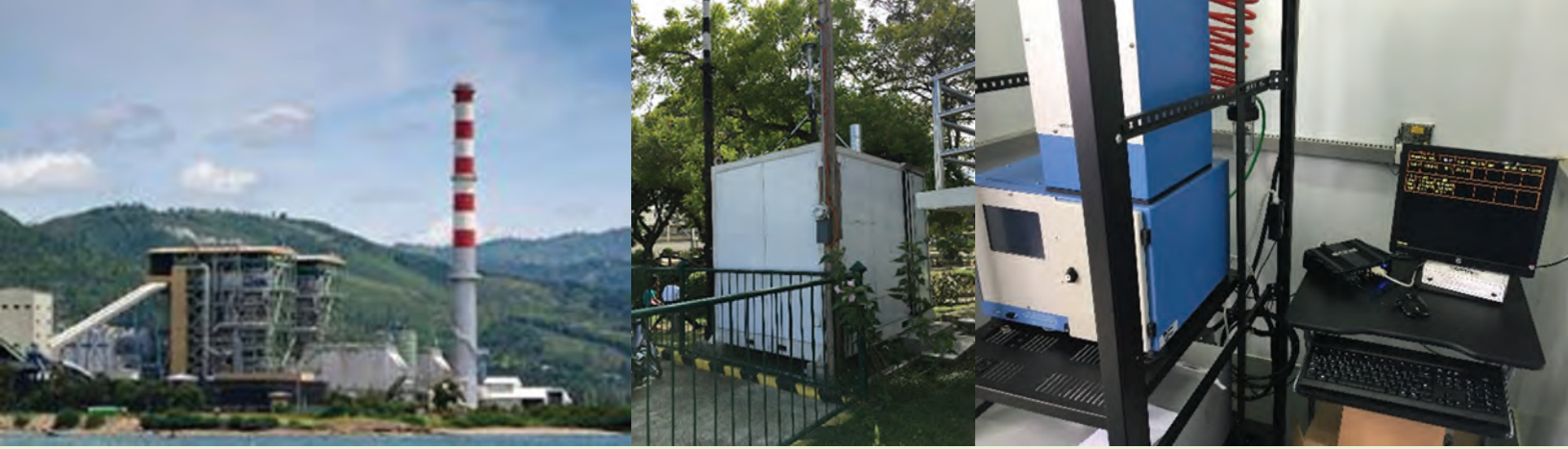
left-right: KSPC power plant; air quality monitoring station in Naga City; and air quality monitoring equipment within the station in Naga City (photos by CRP/OCR).
