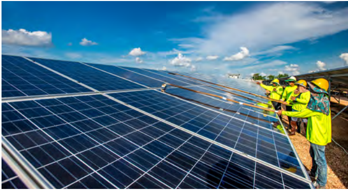
Maintenance crew clean solar panels at the Sunny Bangchak solar farm in Thailand. The plant is part of ADB's support for sustainable energy infrastructure in Southeast Asia.
