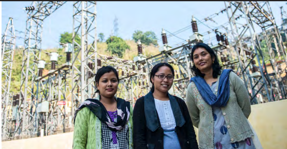
The Narangi Substation near Guwahati in northeastern India is managed by an all-woman team. The 132-kilovolt substation was commissioned in 2009 with ADB assistance.
