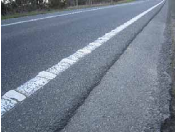
Tactile edge lines have been proven to reduce run-off-road incidents. They are best used in combination with sealed shoulders.
