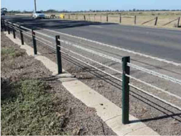
There are several approved wire rope safety barriers in use. They are the most forgiving of the three groups of barriers.
