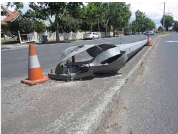
Impact-absorbent poles (such as this one which has been struck) help to minimize injuries to the vehicles' occupants.
