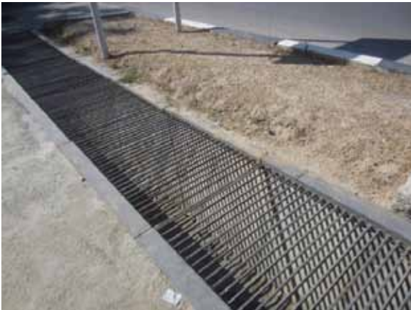
Covering drains within the clear zone can give a smooth drivable and more forgiving area.
