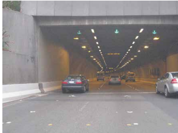
Rigid barriers (concrete) do not deflect, and are well suited where width is limited and deflections cannot be tolerated.
