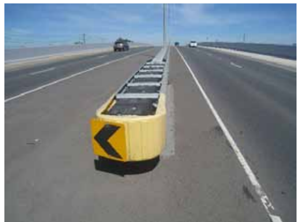
Impact attenuators come in various sizes to accommodate different cross-sections, as well as different speed environments.
