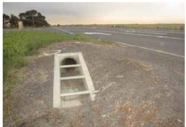
A type 1 drivable end wall is suitable for shielding the ends of pipes parallel to the road.
