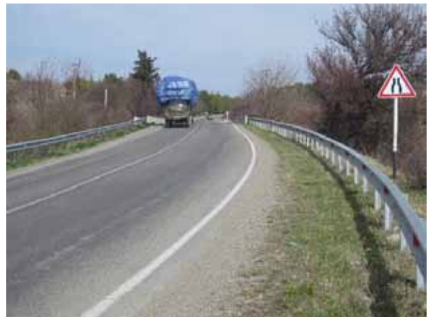
Semirigid barriers have been widely used for decades. They deflect by up to 1 meter when struck. Therefore, they should be at least 1 meter from the hazard they are shielding, and offset by (at least) 4 meters from the road (if the cross-section permits) to allow safe stopping.
