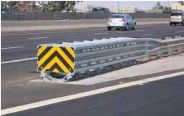
There is a variety of types of impact attenuators. Use only approved types.
