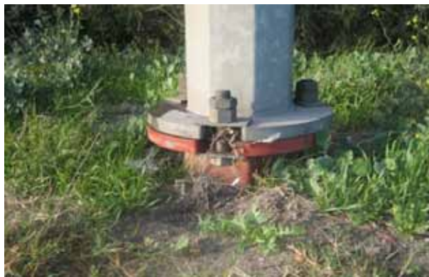
Slip base lighting columns are suitable for use in high-speed areas (80 kilometers per hour and above) where there are few pedestrians and little parking.
