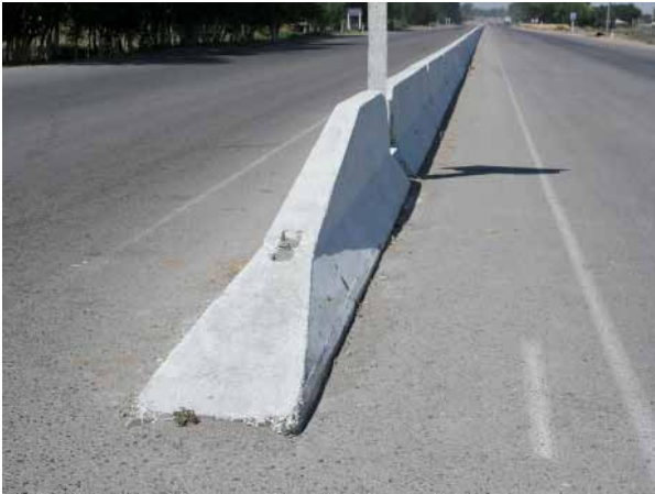
Turned down (or ramped) terminals should not be used on the approach end of barriers in high-speed environments as they tend to launch an impacting vehicle.
