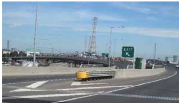
Impact attenuators are well-suited for shielding rigid barrier ends in confined and heavily trafficked locations.
