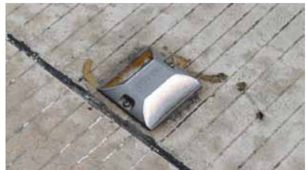
An example of a unidirectional raised reflective pavement marker
