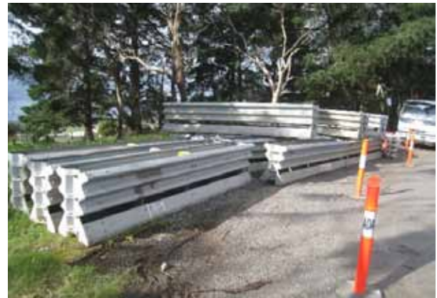
There are portable semirigid barriers that have been approved for use at road work zones. They are recommended for use in work zones.
