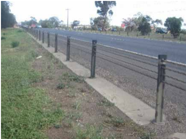
Flexible barriers (wire rope safety barriers) are a proven and safe type of barrier. They can deflect by 2 meters (or more) when struck.
