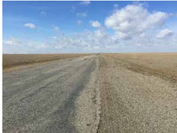
This CAREC highway crosses a large desert. It has wide open and flat roadsides, which provide a good level of roadside safety here. The most obvious safety improvement here would be to include delineation and paved shoulders to keep vehicles on the road.
