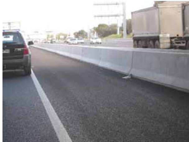
Rigid barriers allow high containment levels to be attained within narrow cross-sections, while (in this photo) still providing sufficient space for a wide inner shoulder.
