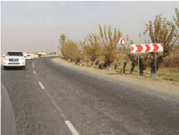
This hazard marker is a standard sign, but it is installed in a nonstandard location. The inside of the curve is not the correct place for such markers. They are to be placed on the outside of curves.
