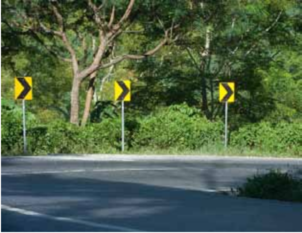
Chevron alignment markers have been proven to assist drivers to safely negotiate substandard curves. Their consistent use across the CAREC highway network is encouraged.
