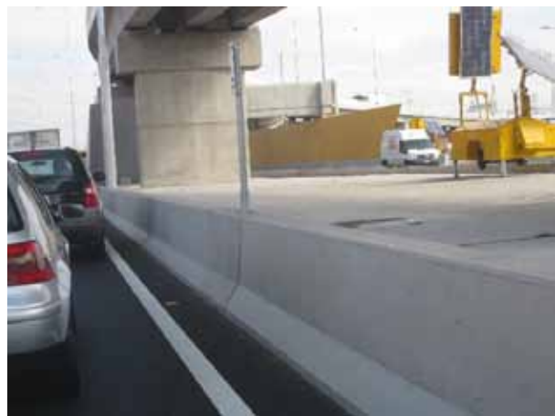
Concrete barriers can be cast in place, or precast and then installed. In complex highway structures, including major interchanges, it is common to cast the concrete barrier as an integral part of the structure.
