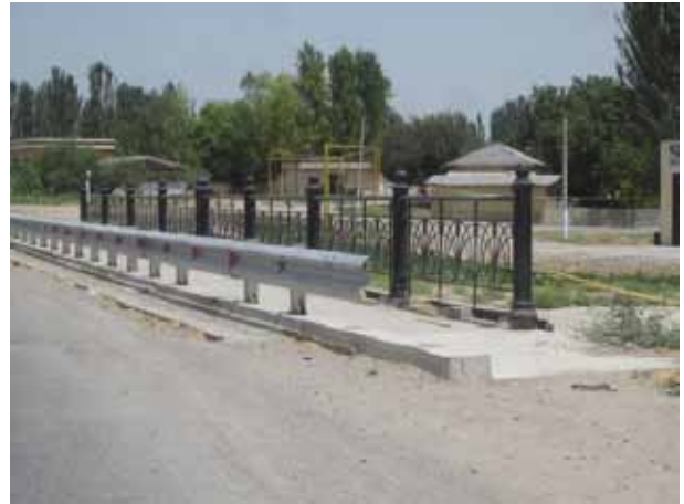
Failing to install a terminal is an unsafe practice. Barrier should not be installed or retained like this as the horizontal rail can easily spear an errant vehicle.
