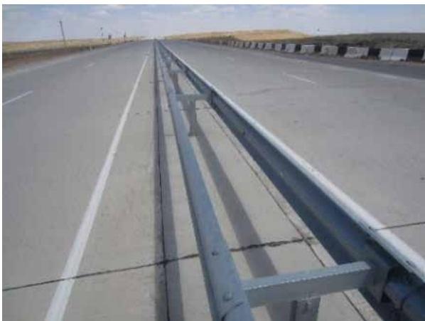
Semirigid barriers (guardrail) are perhaps the most common type of barrier along CAREC highways. They typically deflect by up to 1 meter when struck.
