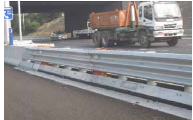
There are several products that close median openings, provide good containment levels, and still permit ready access by authorities during an emergency.
