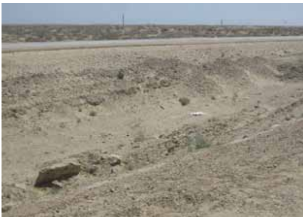
The highway has been designed to high geometric standards. The median has been graded for natural drainage in the desert environment.
