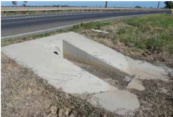
A type 2 drivable end wall is suited for safeguarding the ends of cross culverts.
