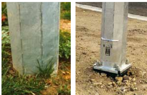
Impact-absorbing lighting columns are suitable for low-speed areas (less than 80 kilometers per hour) where there may be more pedestrians and more parking nearby.
