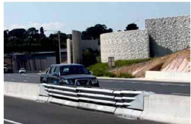
These products can be winched open by an authorized person, and traffic can pass safely from one carriageway to the other during an emergency. It should remain firmly closed at all other times.
