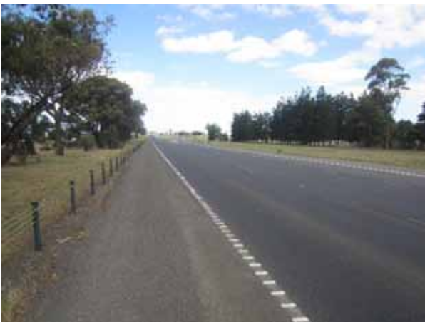
Tactile edge lines alert fatigued or distracted drivers that they are drifting off the highway.
