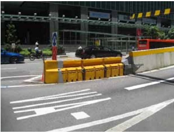
There are several impact attenuators approved for use in advance of temporary rigid barriers at work sites.
