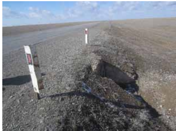
Although there is much flat roadside, care needs to be taken with man-made structures such as culverts (in the photo) and bridges. We can never be sure where or when a vehicle will leave a road.
