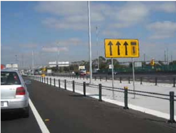
In designing a wire rope safety barrier system, always remember to provide adequate offset between the barrier and the hazard to accommodate the barrier deflection. Flexible barriers can deflect by 2 meters or more.
