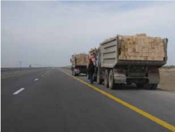
Sealed shoulders also provide a place where vehicles can stop in emergencies (to check loads, or during medical emergencies).
