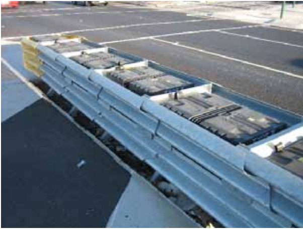
Some impact attenuators have crushable cells inside the steel structure to absorb much of the impacting energy. Lower-cost models have alternative systems.
