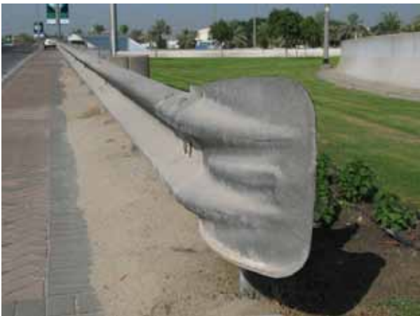
"Fish tail" terminals present a spearing risk and should not be used on CAREC highways.
