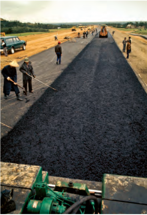
Yangmei freeway project in Taipei, China, 30 March 1970.
