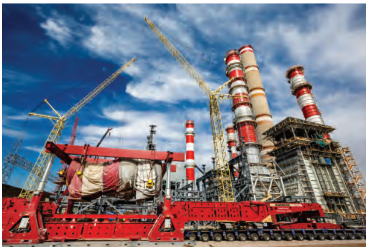
ADB is helping Uzbekistan boost the efficiency of its electricity supply by building an 800-megawatt combined cycle gas turbine power plant. Located 440 kilometers southwest of Tashkent, the new facility will increase energy efficiency through clean power generation, 20 April 2010.
