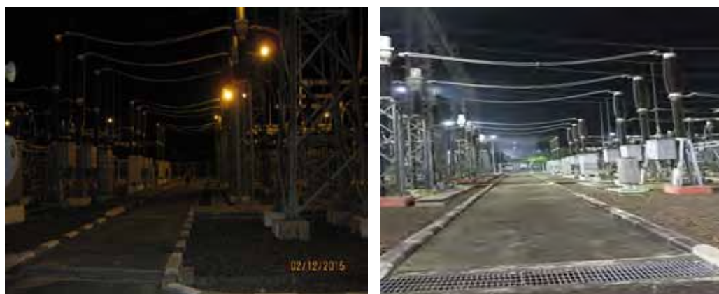
Figure 6: Lighting Conditions at Cilegon Substation Before and After the LED Retrofit
