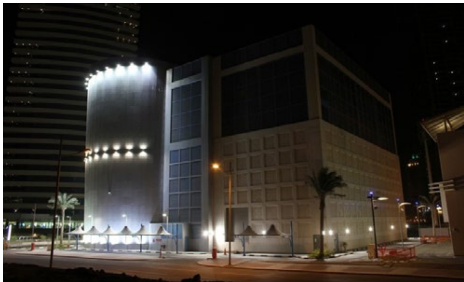
Figure 18: District Cooling Plant in Qatar
