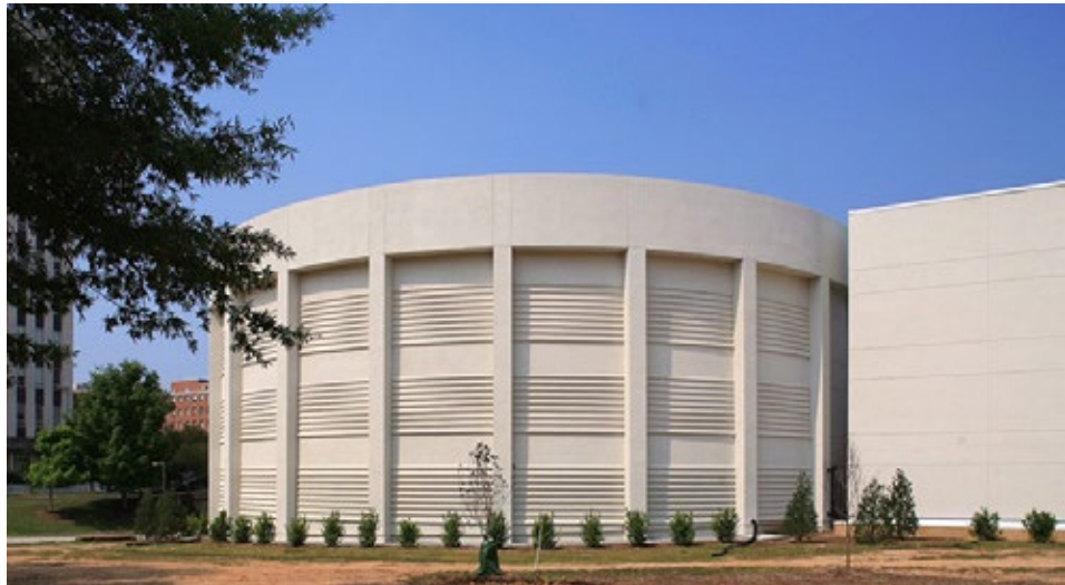
Figure 6: Thermal Energy Storage in Raleigh, North Carolina, US
